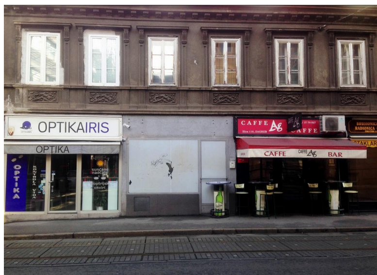
Fig. 9: A view on the Ilica St. 116 micro-location from across the street during a visit in November, 2016
