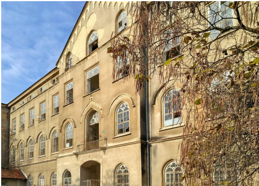
Picture 4. Yard building facade
