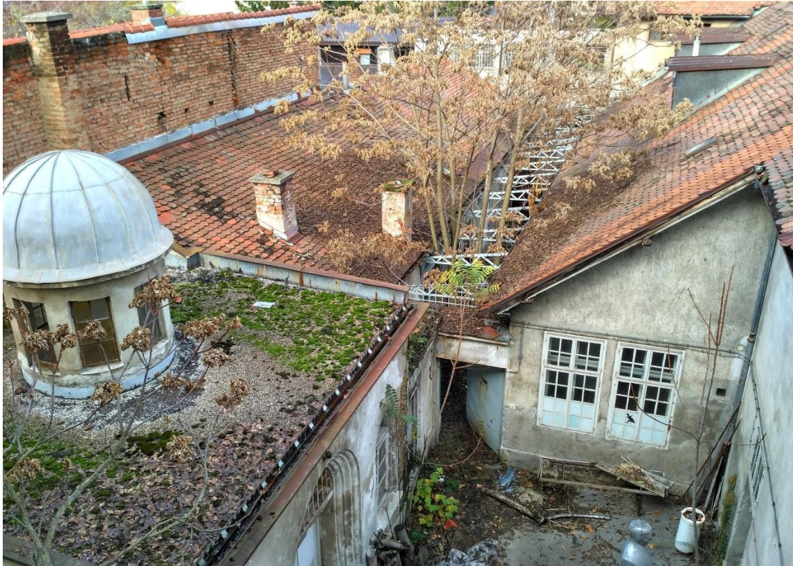
Picture 2. View on the junction building
